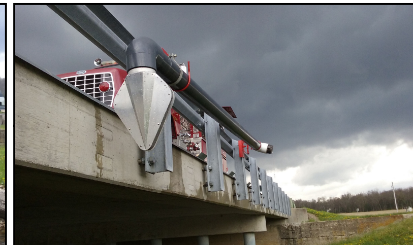
Hydrant in stowed position
