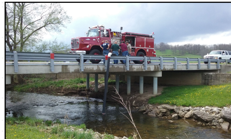
Hydrant deployed for drafting
